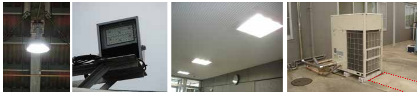
佐野事業所の倉庫や屋外の水銀灯をLED化 At the Sano site, warehouse and outdoor mercury lamps were changed to LEDs.
