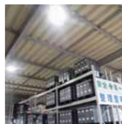
新倉庫 LED LEDs in the new warehouse
