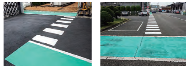
Pedestrian paths installed in the plant
