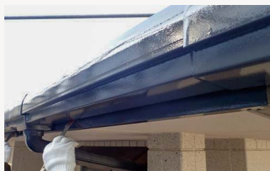
Brush-painted eaves gutter
