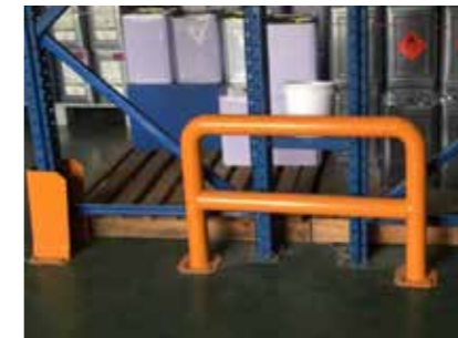
倉庫内防護柵設置 Protective barrier in the warehouse
