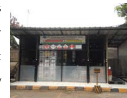
Temporary storage site for hazardous materials before disposal, installed according to relevant law
