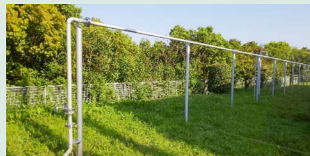
Aboveground installation of piping that was previously buried in the ground
