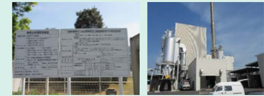
Facilities of waste treatment companies
