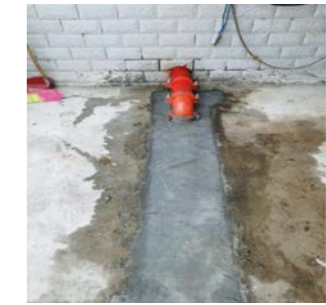
Outdoor underground piping after repair
