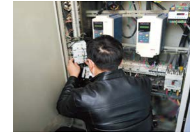
Inspection of operational conditions
