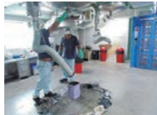
Drill against a leak from the lower part of the tank
