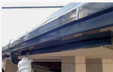
Brush-painted eaves gutter
